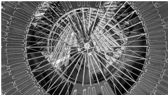
Fig. 4. Conical roofing of MSVU silo with a diameter of 33m "Lubnymash"
