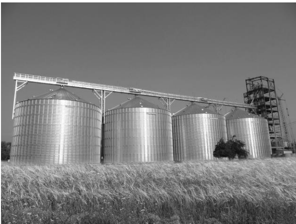
Fig. 1. General view of the vertical steel cylindrical containers of "Lubnymash" ( https://lubnymash.com/ )
