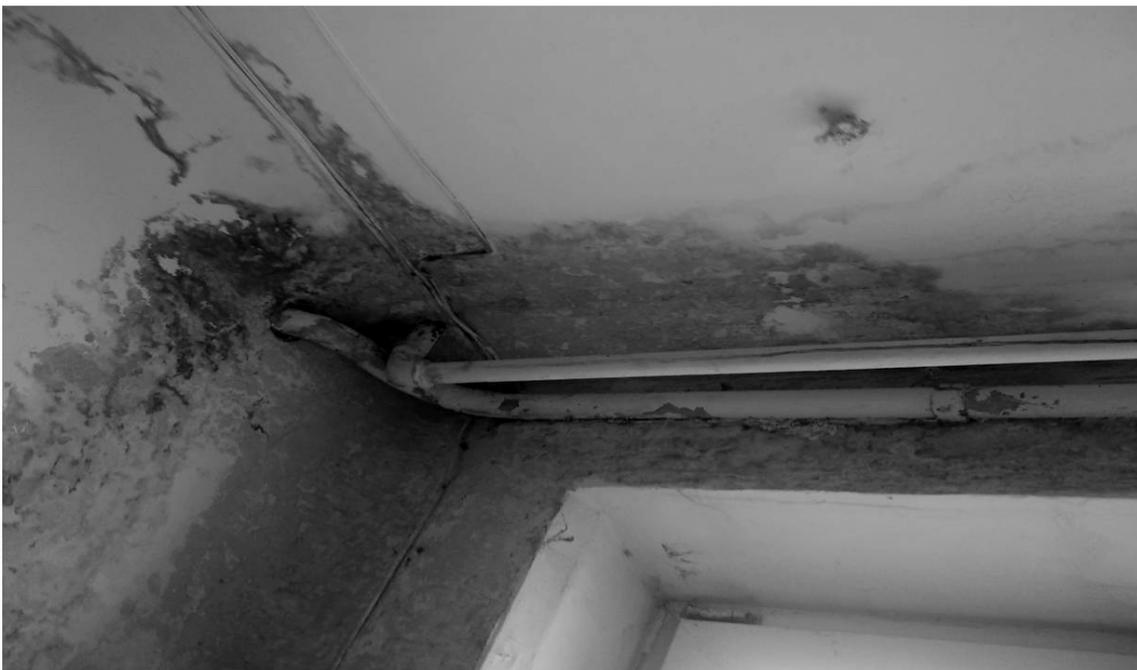
**Fig. 2.** The microbiological corrosion in residential building
