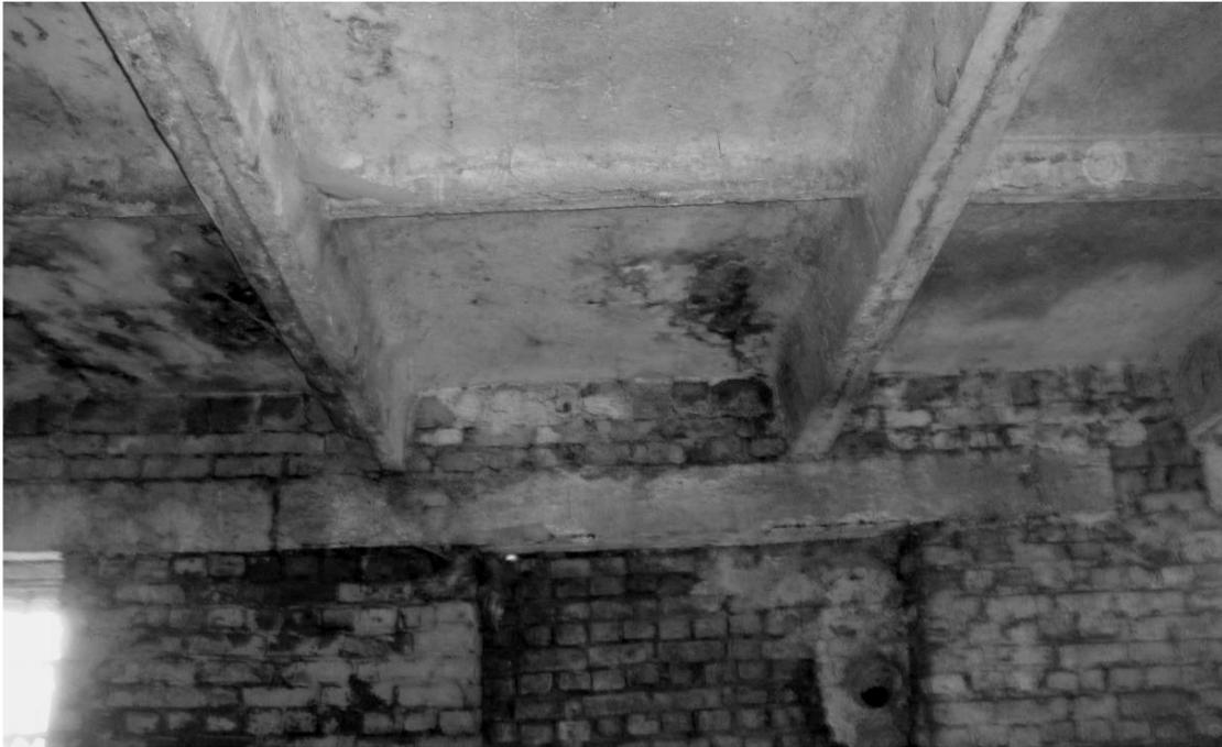
**Fig. 1.** The microbiological corrosion in industrial building
