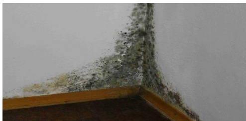
Figure 5 – Biological corrosion in animal farm
