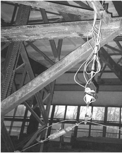
Fig. 8. The insulator string's general view
