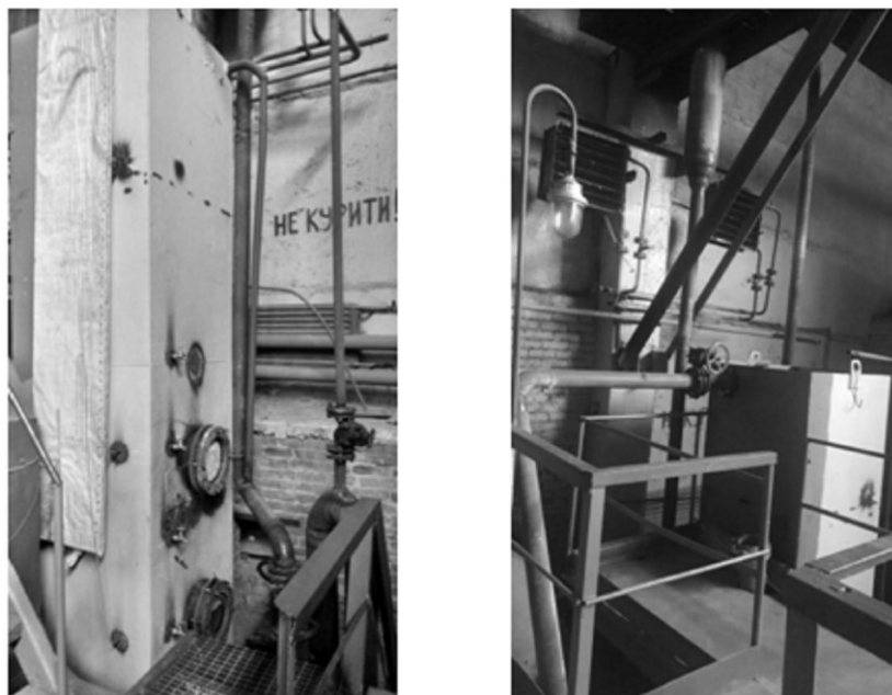
Fig. 3. Photos of industrial experimental plant for research of softening process
