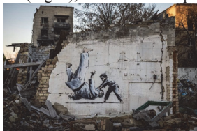
Fig. 1. Graffiti on the wall of the destroyed boiler house in Borodianka as of 11.11.2022. (Photo by Ed Ram)
