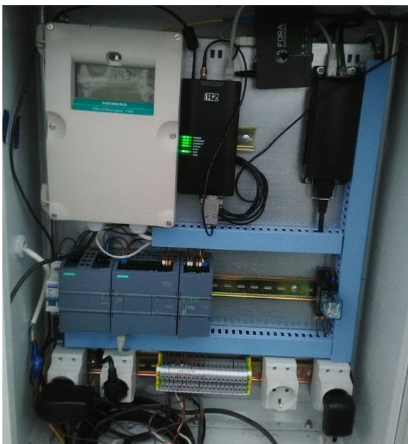
Fig. 1. Exterior view of the mounting container GIS-Dniester
