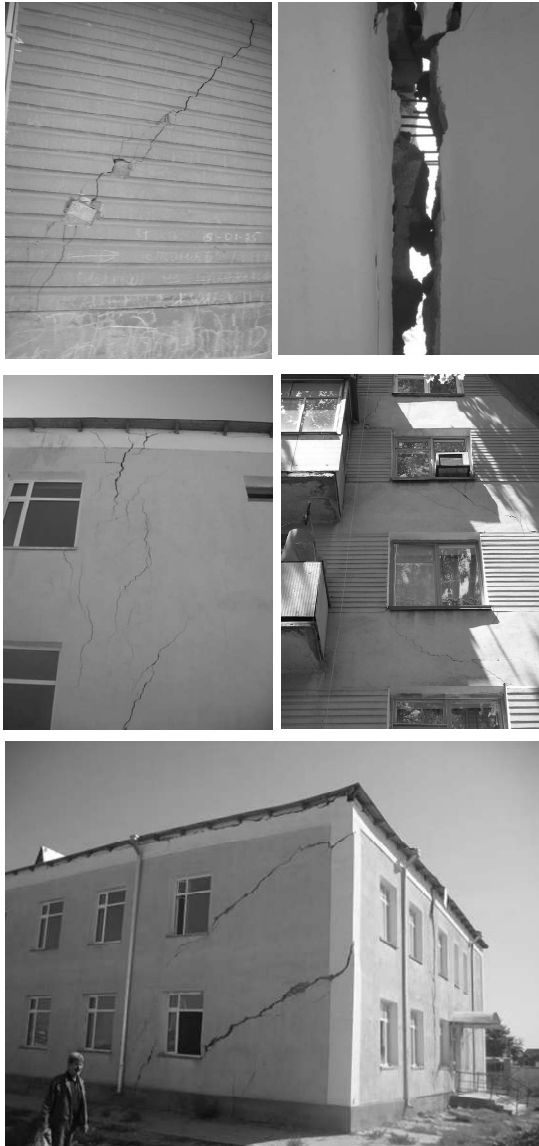
Fig. 1. Damages of buildings bearing walls in seismic areas by substantial differential settlements of soil base
