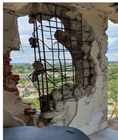
Fig. 5. Pylon hit by a projectile. Photo by V. Nuzhnyi
