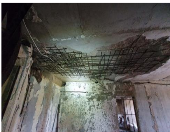
Fig. 12 Complete destruction of the working reinforcement in the ceiling after prolonged exposure to fire. Photo by V. Nuzhnyi
