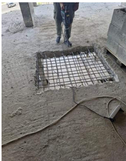
Fig. 10 Cleaning damaged concrete after a pinpoint hit by a small-caliber projectile. Photo by V. Nuzhnyi
