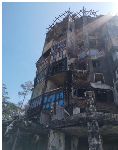
Fig. 3 Exterior view of a section of a building with a monolithic reinforced concrete frame that was damaged during hostilities. Photo by V. Nuzhnyi
