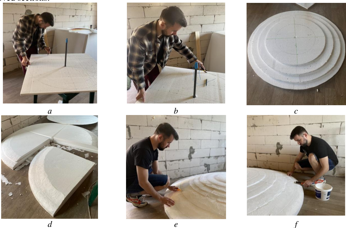
Fig. 5. Procedure for creating polystyrene formwork: a) manual marking of individual polystyrene sheets; b) basic cutting of fragments with a utility knife; c) general view of blanks before edge trimming; d) blanks after edge trimming; e) shape adjustment after assembling the formwork; f) puttying of seams and joints. Photo by V. Tenensku
