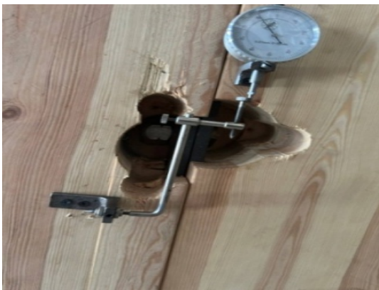
Fig. 15 Failure of bolt M20 and enlarged hole milled in the timber for bolts M24. Photo by Andrii Bidakov
