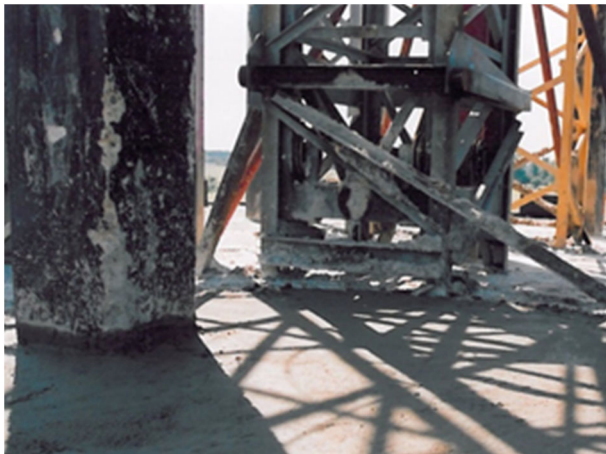
Fig.5. The top plate after concrete casting
